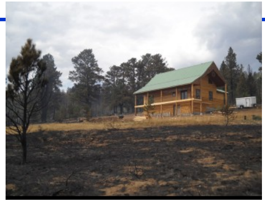
This landowner implemented defensible space zone improvements. The Shepherder Hill fire burned around the structure on all sides.
