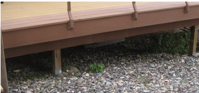
Coarse gravel pad under a deck
