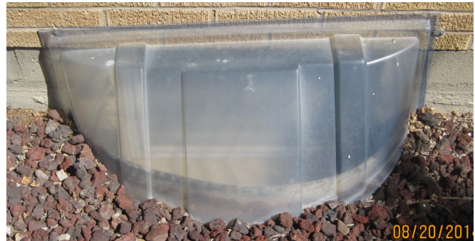
Covered window well and cinder mulch
