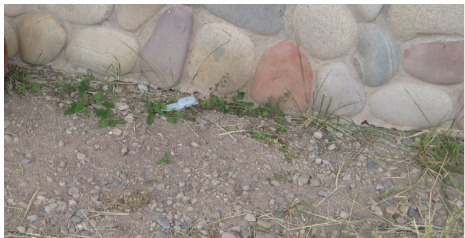
Fine gravel around foundation
