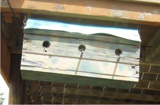
← Great Grandpa made this three-plex birdhouse. It's now filled with grass and twigs that would be quickly ignited by flying embers.
