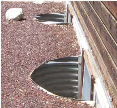
Open window wells. Should be kept clear of leaves and forest litter, or covered.
