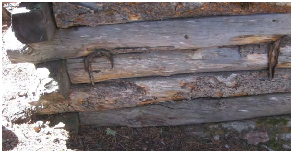
Unsealed rough logs in contact with forest litter, AND with ember trap bark attached. Remove bark, seal the logs & crevices, and keep a three-foot swath cleared to bare mineral soil.
