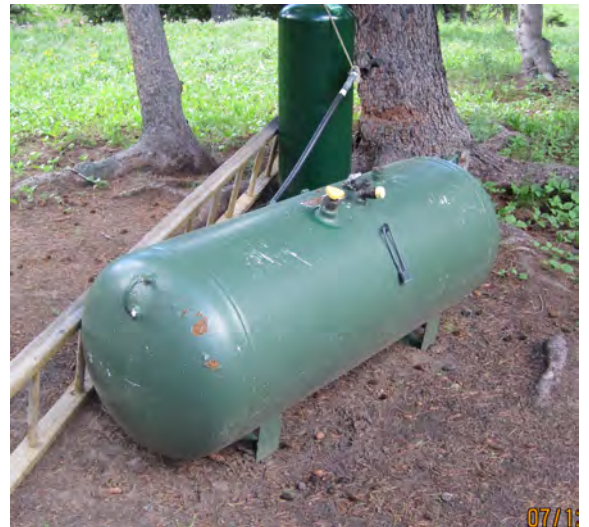
Propane tank is a cleared spot, but with an old wooden ladder leaning against it.
