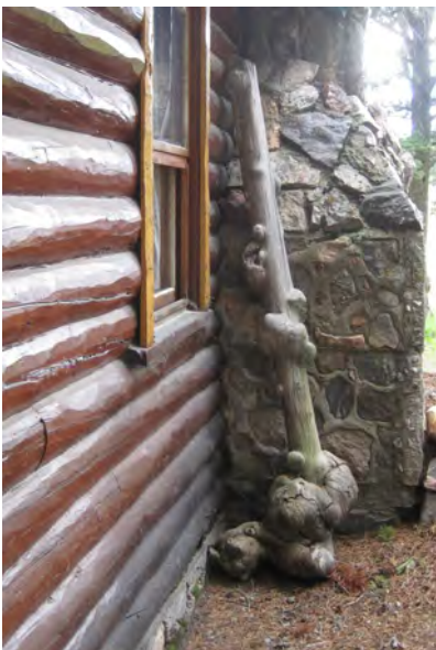
Dry forest litter and "special" dry wood by cabin wall and single-paned window.
