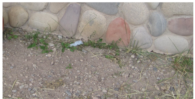
Fine gravel around foundation
