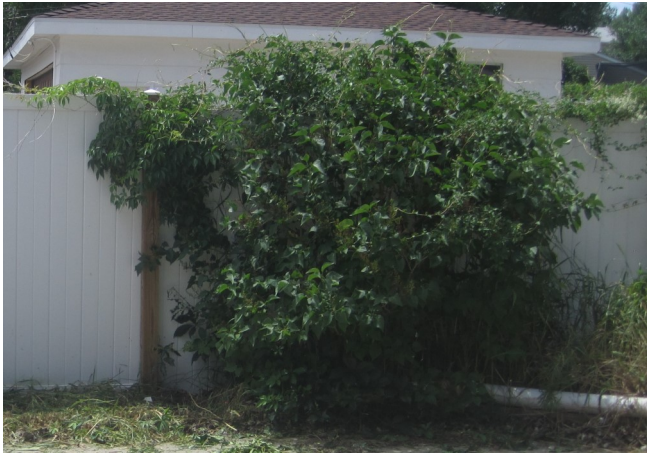
A fence overgrown with vegetation. Would increase the chance of the fence igniting. Keep shrubbery trimmed to three feet from the fence.
