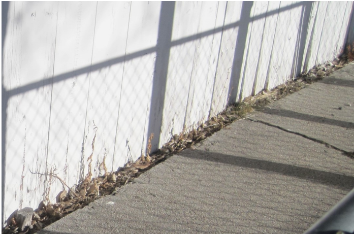
Wooden fence with ember-trapping tinder base.
