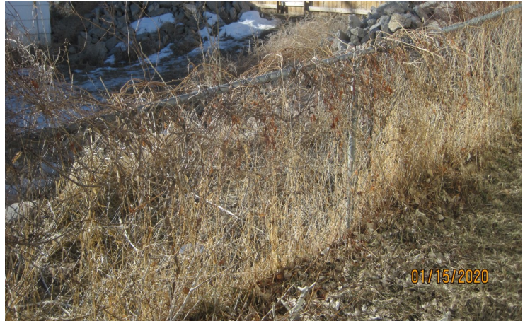
Wire fencing filled with flammable vines. Fire would travel along this metal fence. Removed vines from fence and below it.
