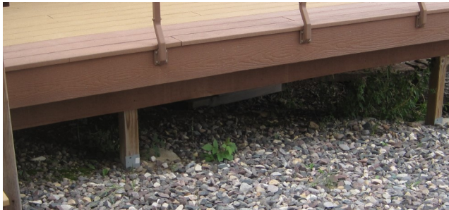
Coarse gravel pad under a deck
